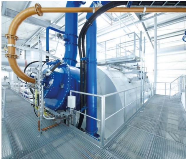
Gas fired industrial boiler for process steam
